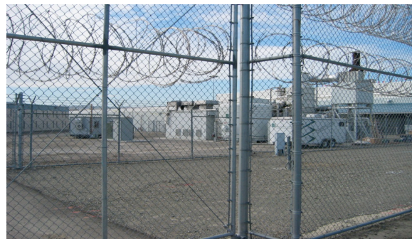
Figure 12 Existing Fuel Cell and Battery Site
