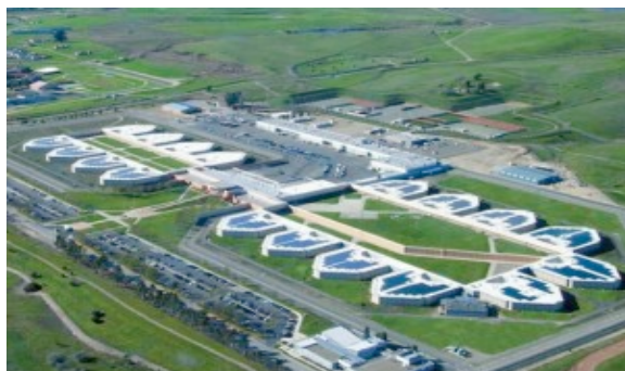
Figure 11 Aerial View of Santa Rita Jail
