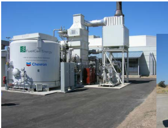
Picture above: 1 MW single direct fuel cell Module at the Santa Rita jail
