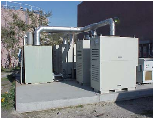
Picture below: Microturbines
