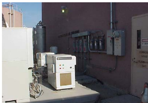
Picture above: Microturbine disconnection switches
