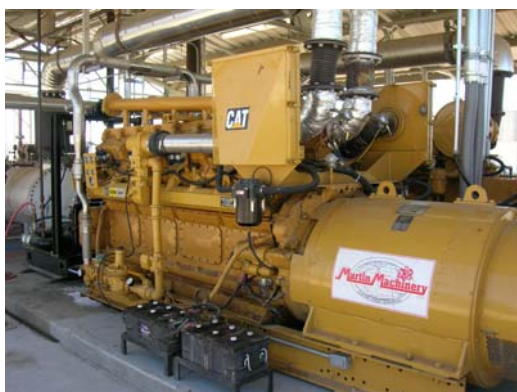
Picture above: 400 kW reciprocating engine
